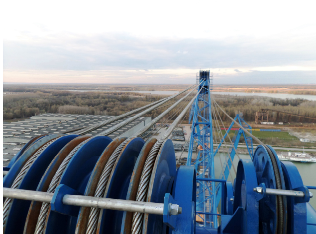
Figure 5 Lattice boom of the crane, view from the top end of the mast
