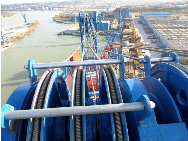
Figure 4 Mast of the crane, view from the top end of the truss arm
