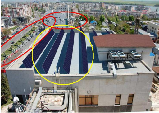
Figure 7 Overview of the hybrid wind / photovoltaic system
