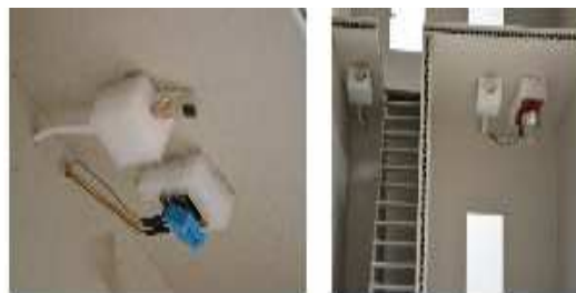
Figure 4 The fire and flood sensors placed on the ceiling
