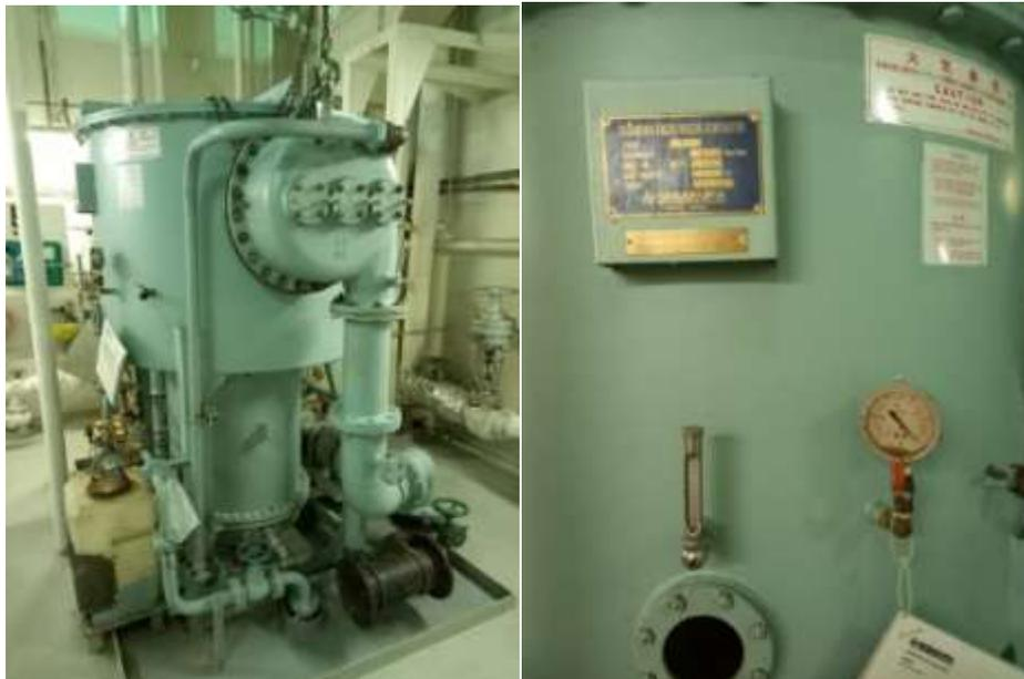
**Fig. 5.1** Freshwater generator SASAKURA KM50
