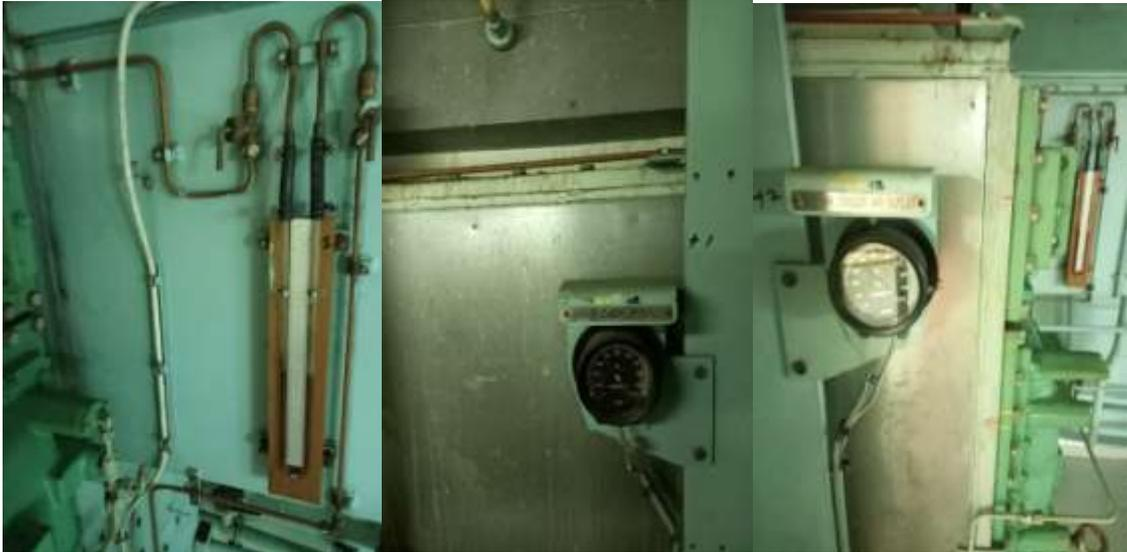
**Fig. 7.1** Turbocharging system measuring points
