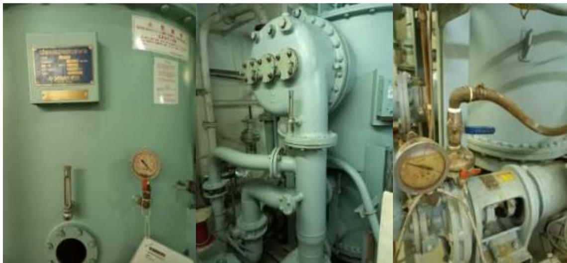
Fig. 7.2 Freshwater generation system measuring points
