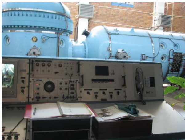
Figure 1 The hyperbaric complex with the wet chamber and the dry chamber
