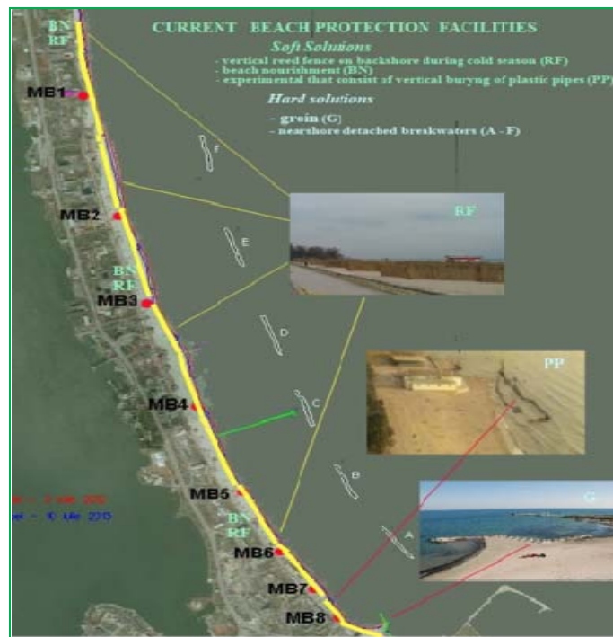
Figure 2 Current beach protection facilities
