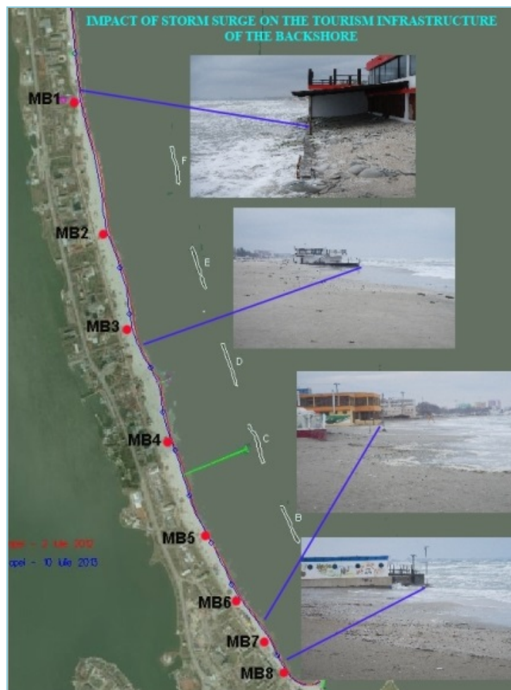
Figure 3 Impact of storm surge on the tourism infrastructure of the beach
