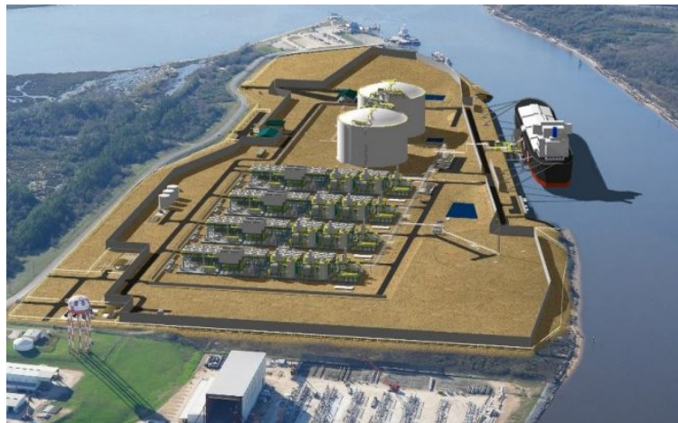
Figure 3 Site for another LNG generation, storage and transport plant
