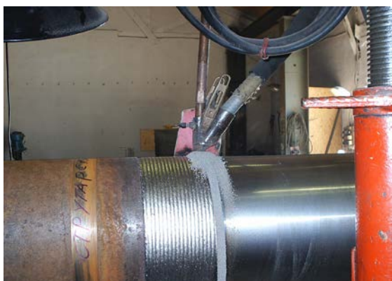
Figure 1 Flux-cored built up welding of the worn-out bearing hub
