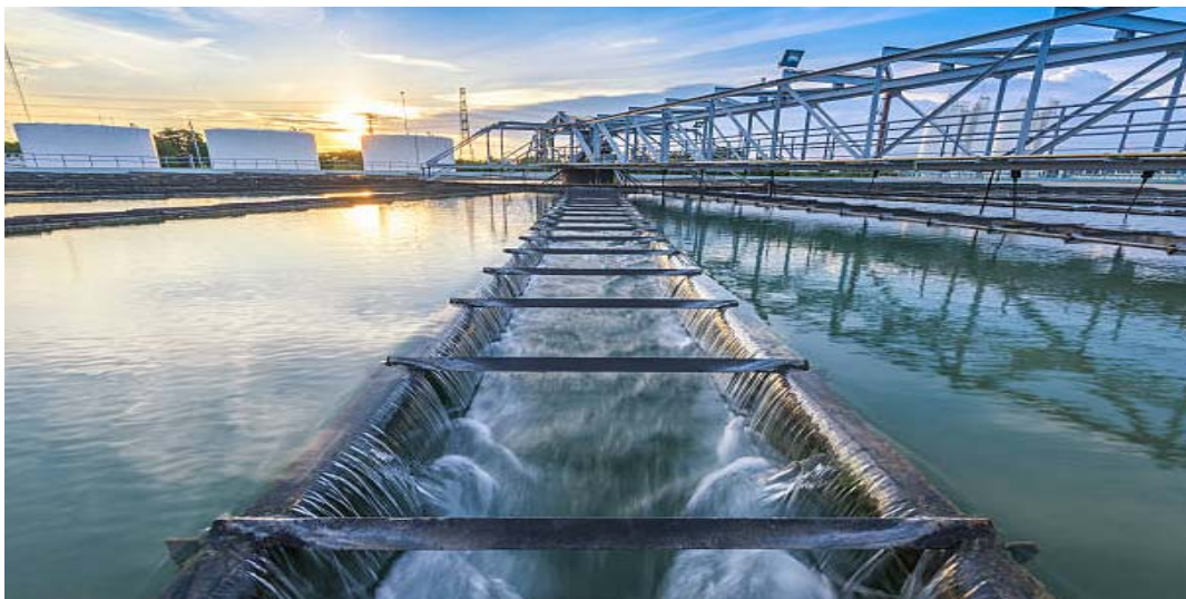
Figure 10 Sewage treatment plant at the quay [9]
