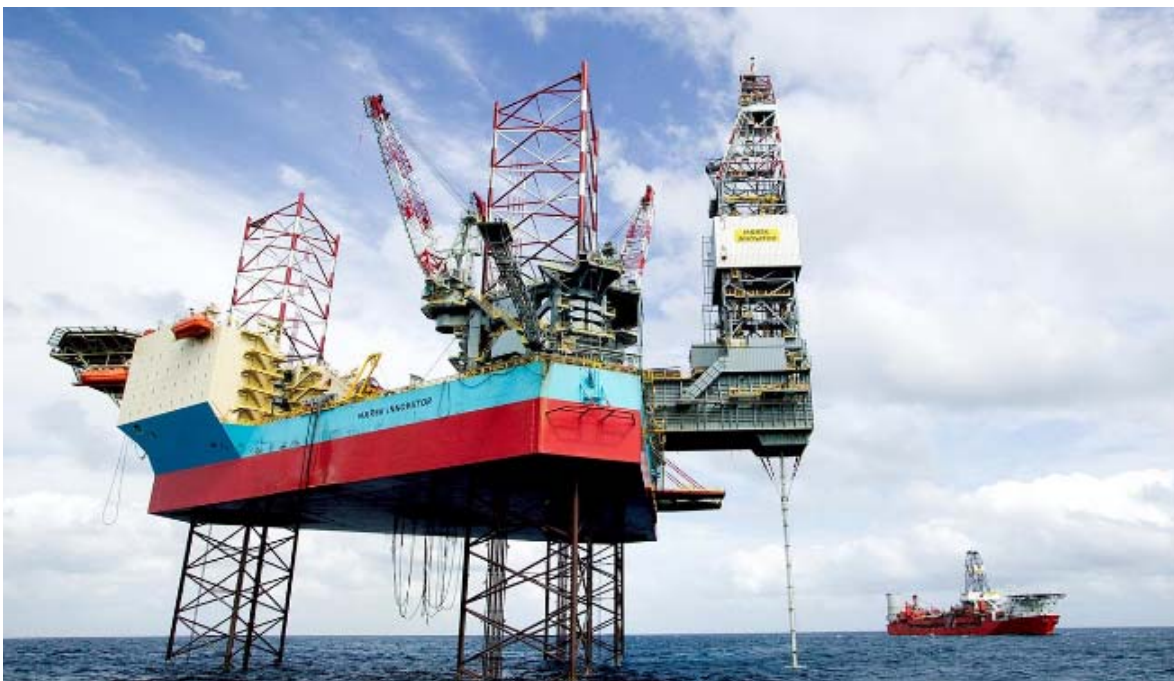
Figure 8 Overview of a Marine Drilling Platform [7]
