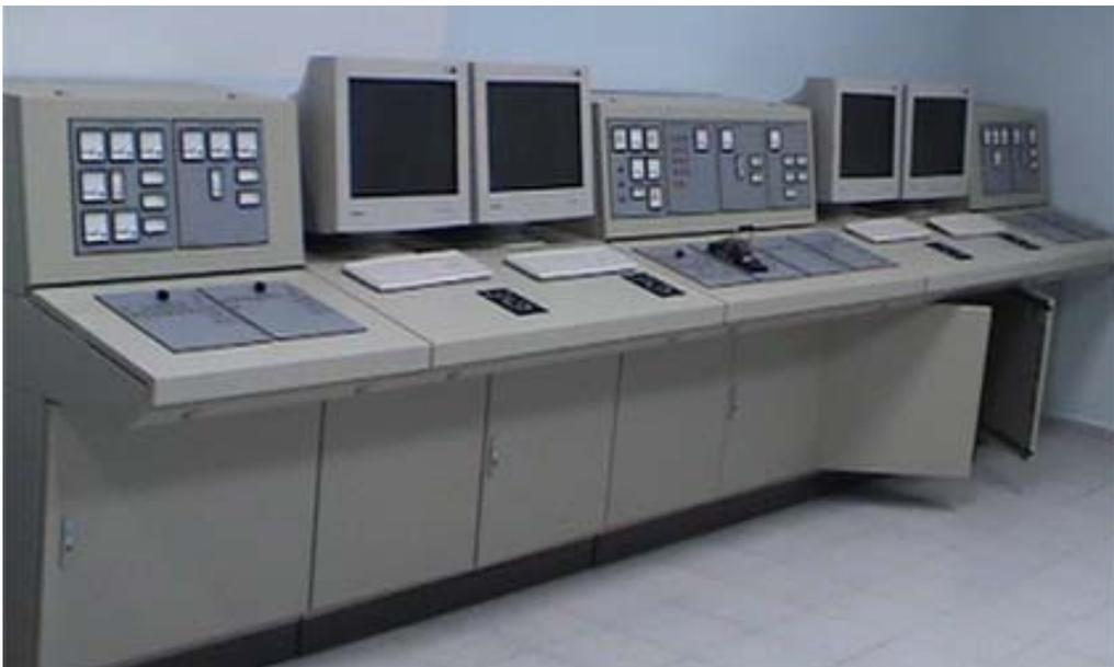
**Fig. 3 Control board of ship power plant consists of panel for main engine control and auxiliary engines control panels.**
